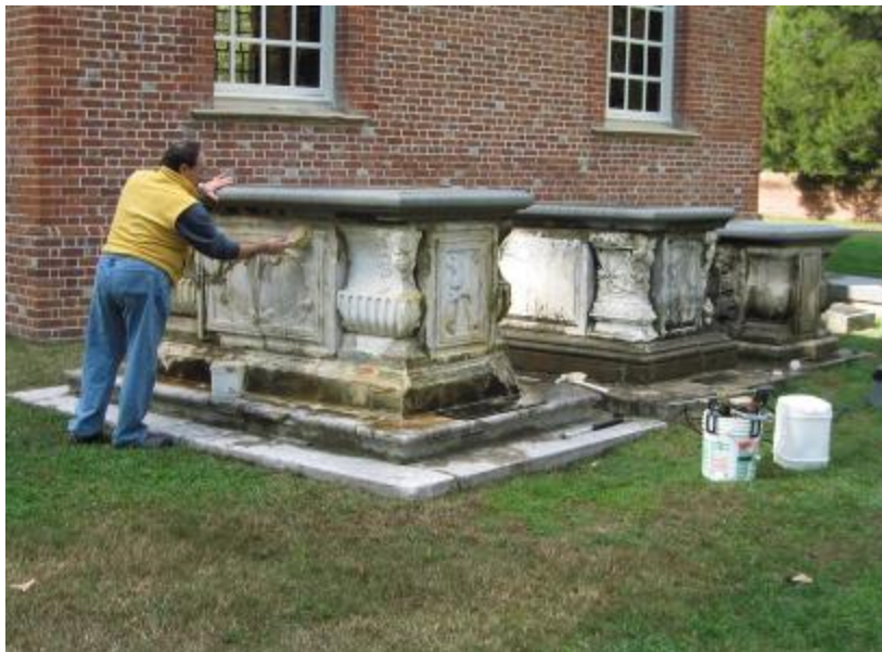
Removal of biological soiling to facilitate inspection, November 4, 2002
