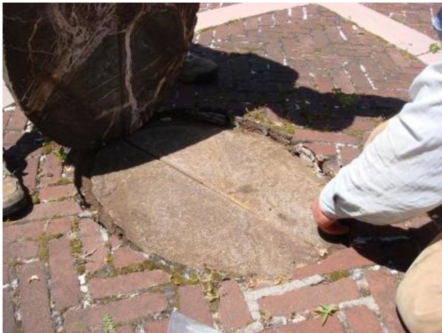
Removal of oval plaque in center of Southwest quadrant to examine setting area. Note stone slab for setting.
