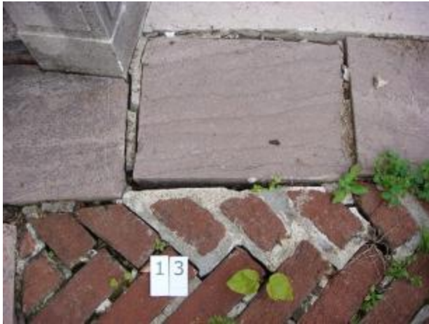
Loose limestone fragment
