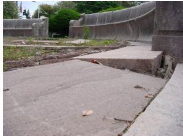
Stone displacement
