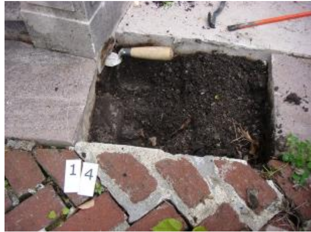
Limestone fragment removed. Note depth of trowel under corner of exedra.
