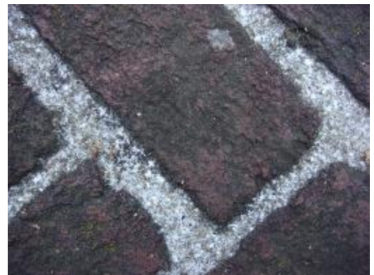
Detail of joints assumed to be original
