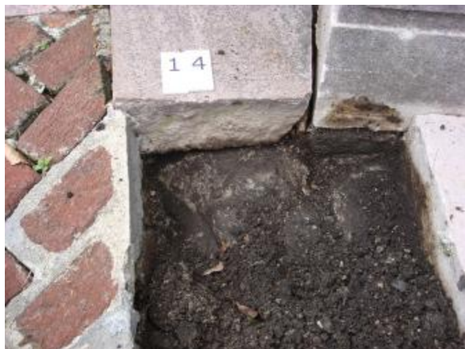
Detail of setting area
