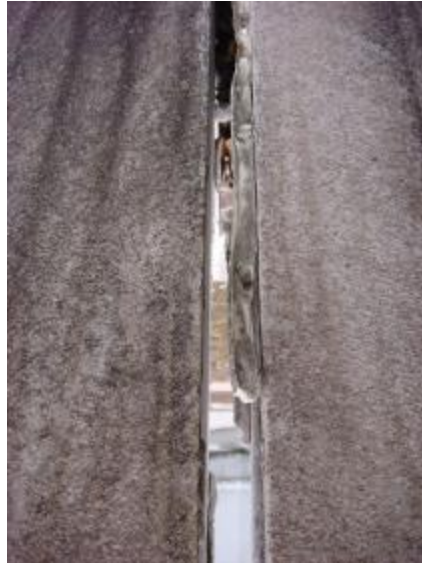
Detail of existing open joints with failed replacement caulking and fibrous backer material.
