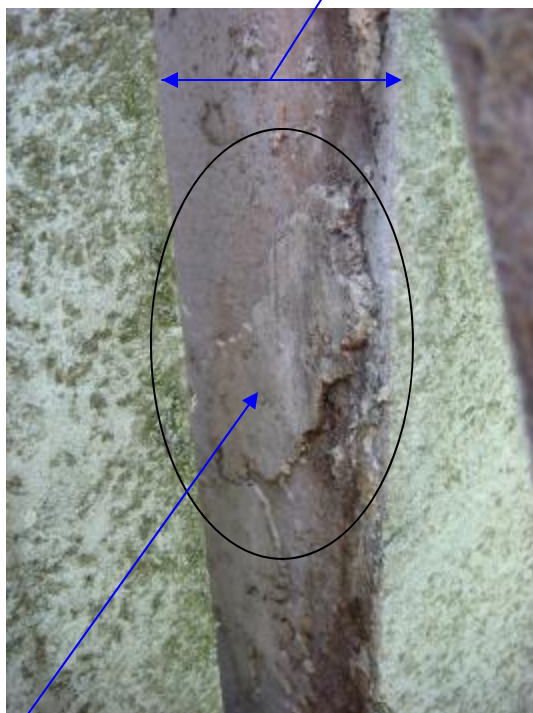
Detail of original thin joint mortar
