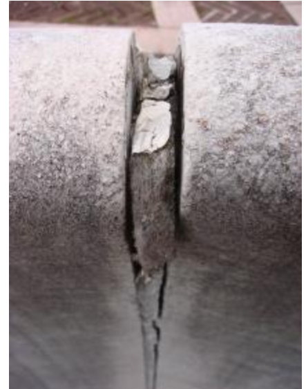
Detail of existing open joints with failed replacement caulking and fibrous backer material.
