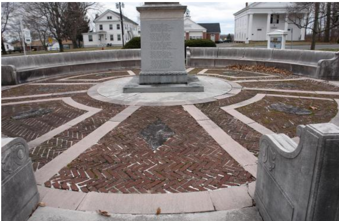
View of pavement from East entrance
