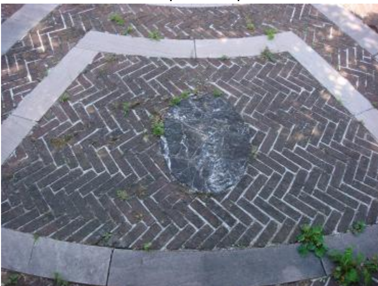
The spacing of the joints and appearance of the mortar in the South-East paving surrounding the oval plaque appears to be original.
