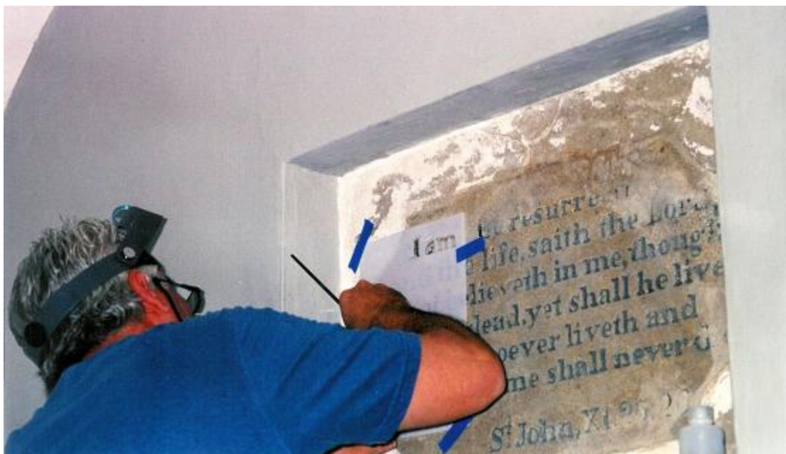
Use of stencils to apply isolating layer.
