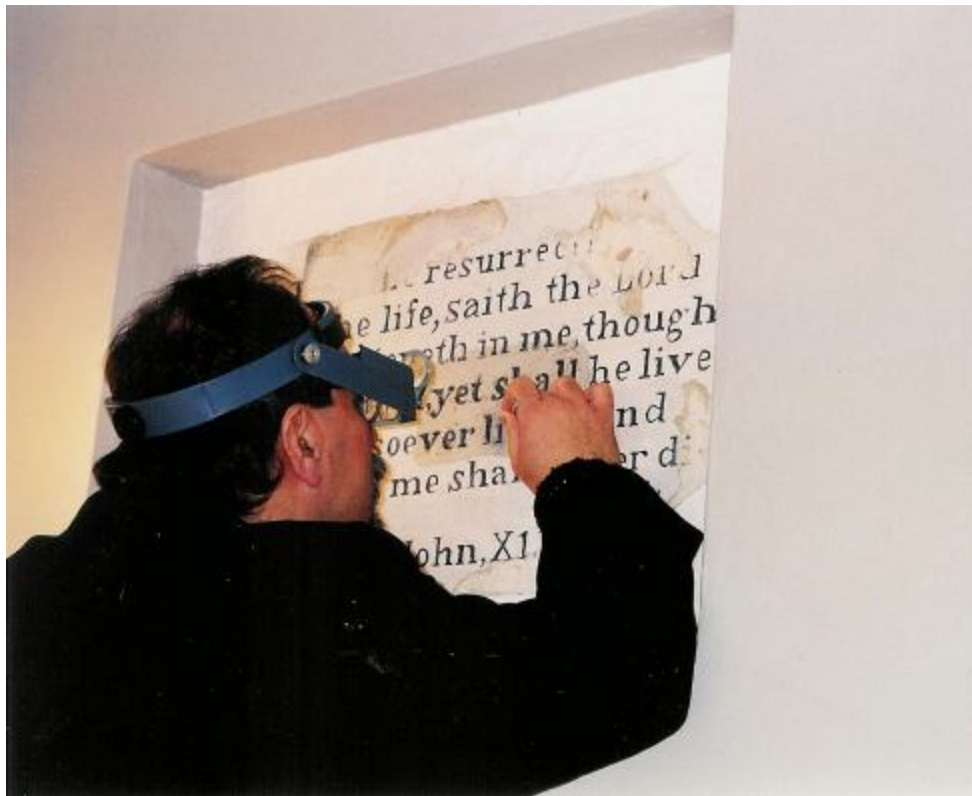
Initial testing of paint stripping.
