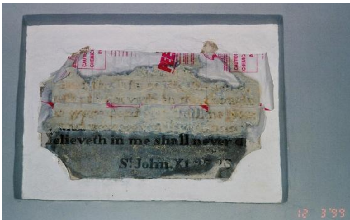
Application of "Peel Away 7" to upper portion of field.
