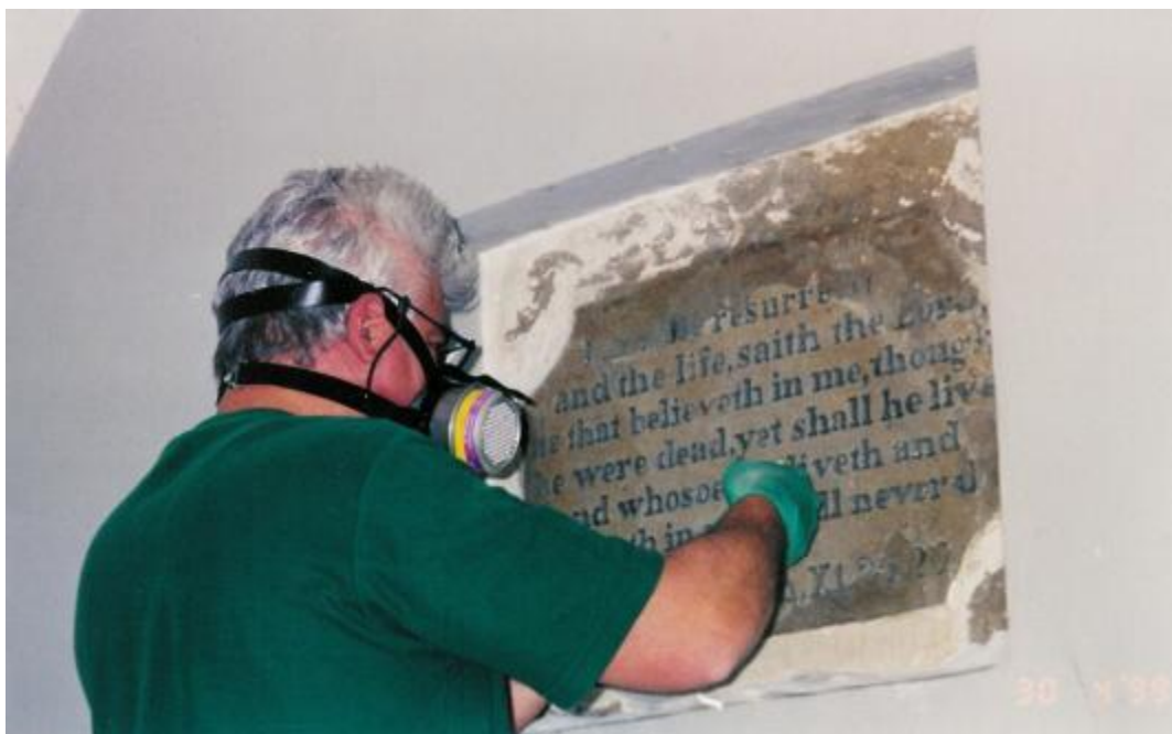
Application of "Conservare OH" consolidant
