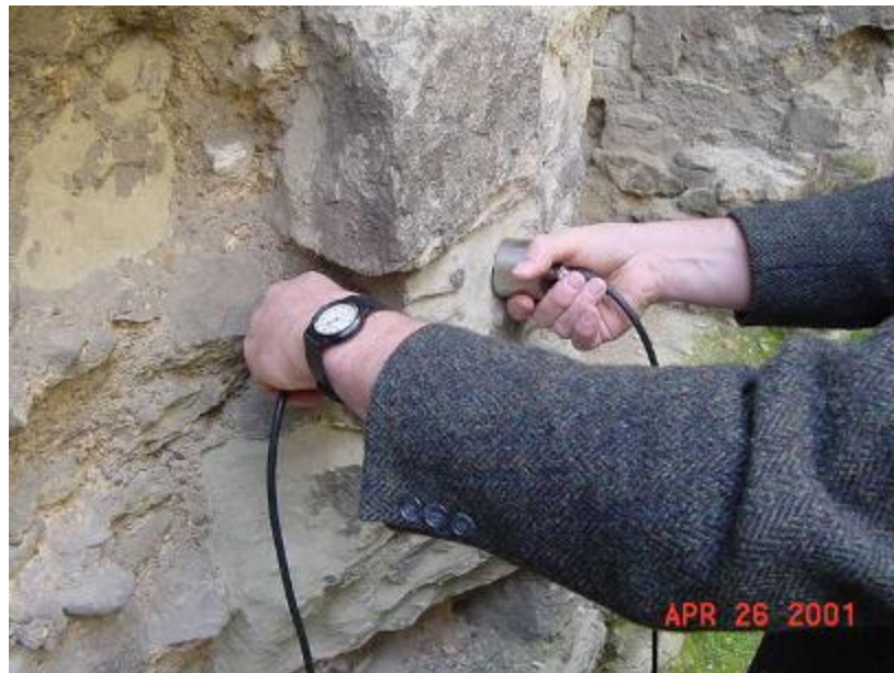
Measuring ultrasonic transit time with PUNDIT
