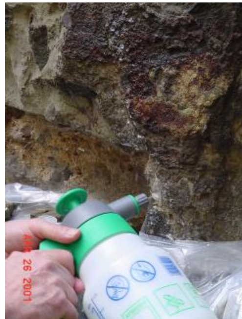
Applying treatment with low pressure spray
