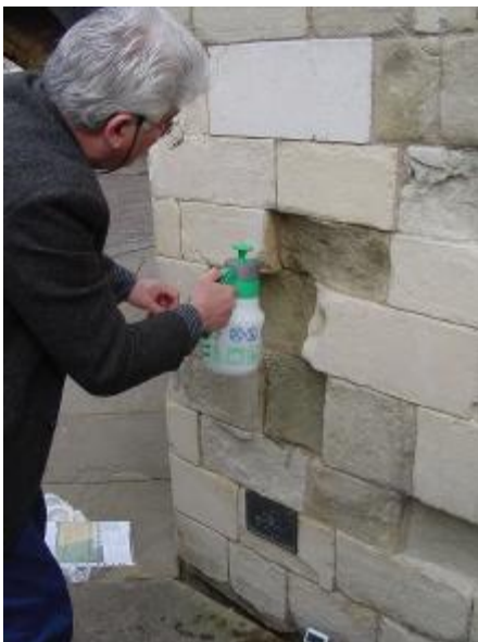
Application of treatment with low pressure spray
