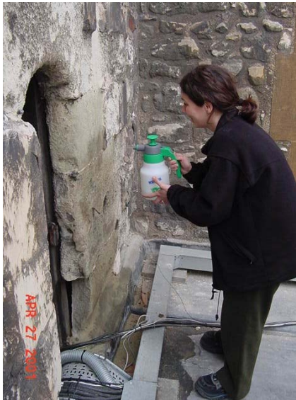
Application of HCT
