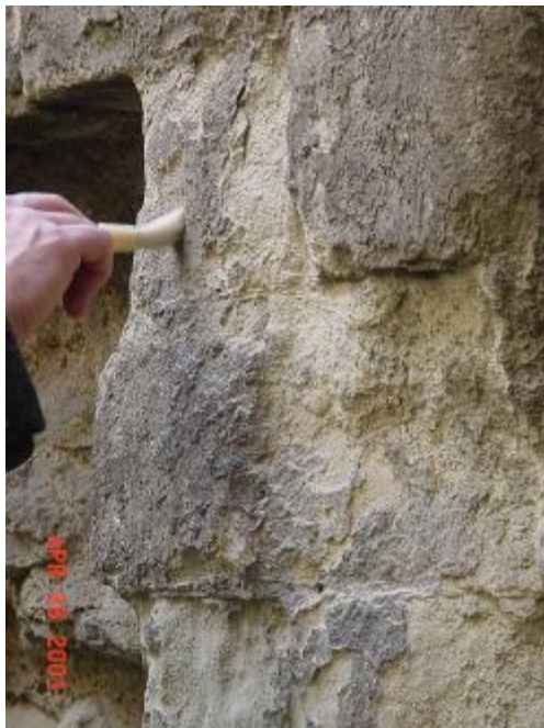
Removing loose surface material by lightly brushing
