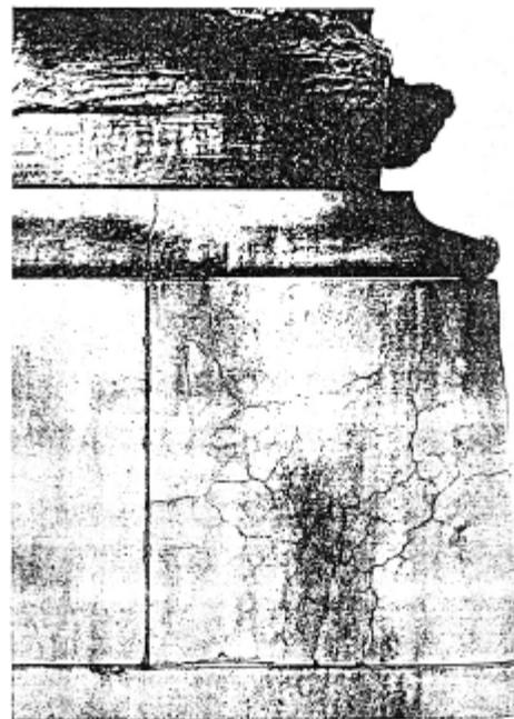
FIGURE 3. Block of badly cracked marble under the north statuary group of the Grant Monument showing the worst condition in this structure.
