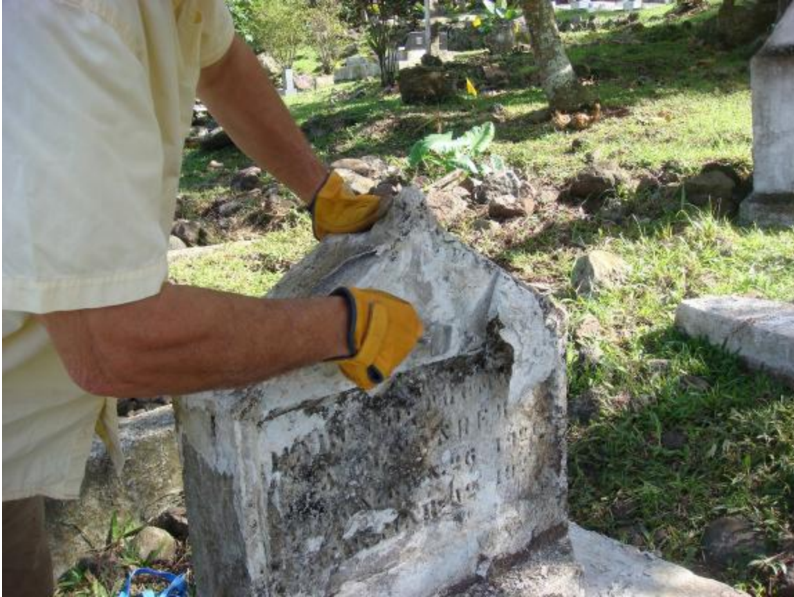
Loose layers of old paint were scraped or peeled off before applying D/2 Biological Solution.
