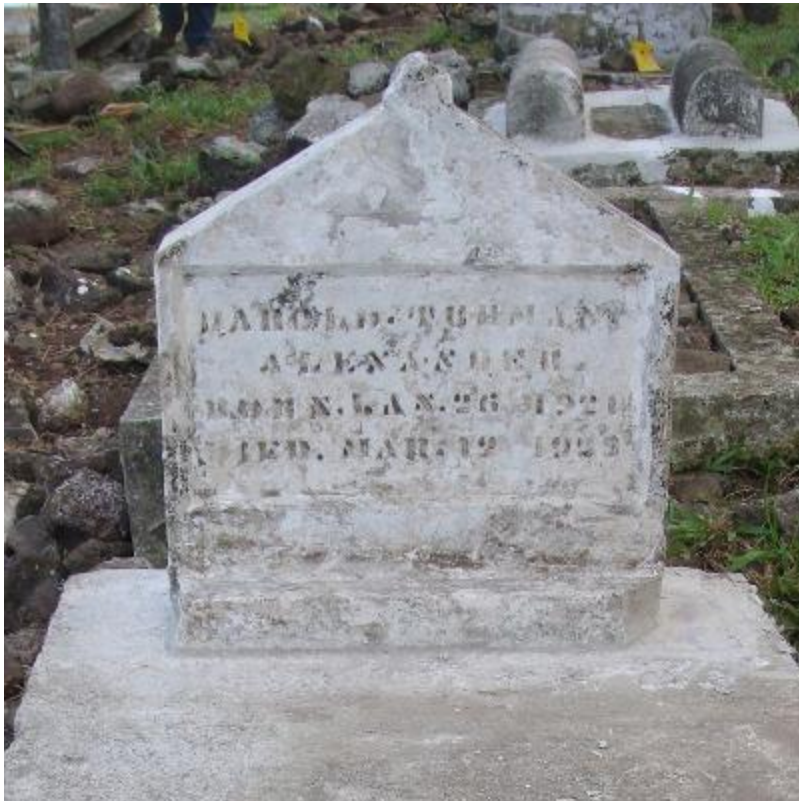
Loose layers of old paint were scraped or peeled off before applying D/2 Biological Solution.
