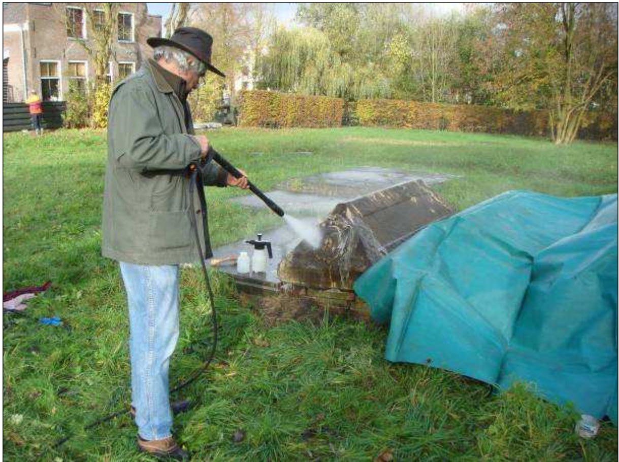
Pressure washing in progress at the nr. 1 stone that has been cleaned with Biowash.
