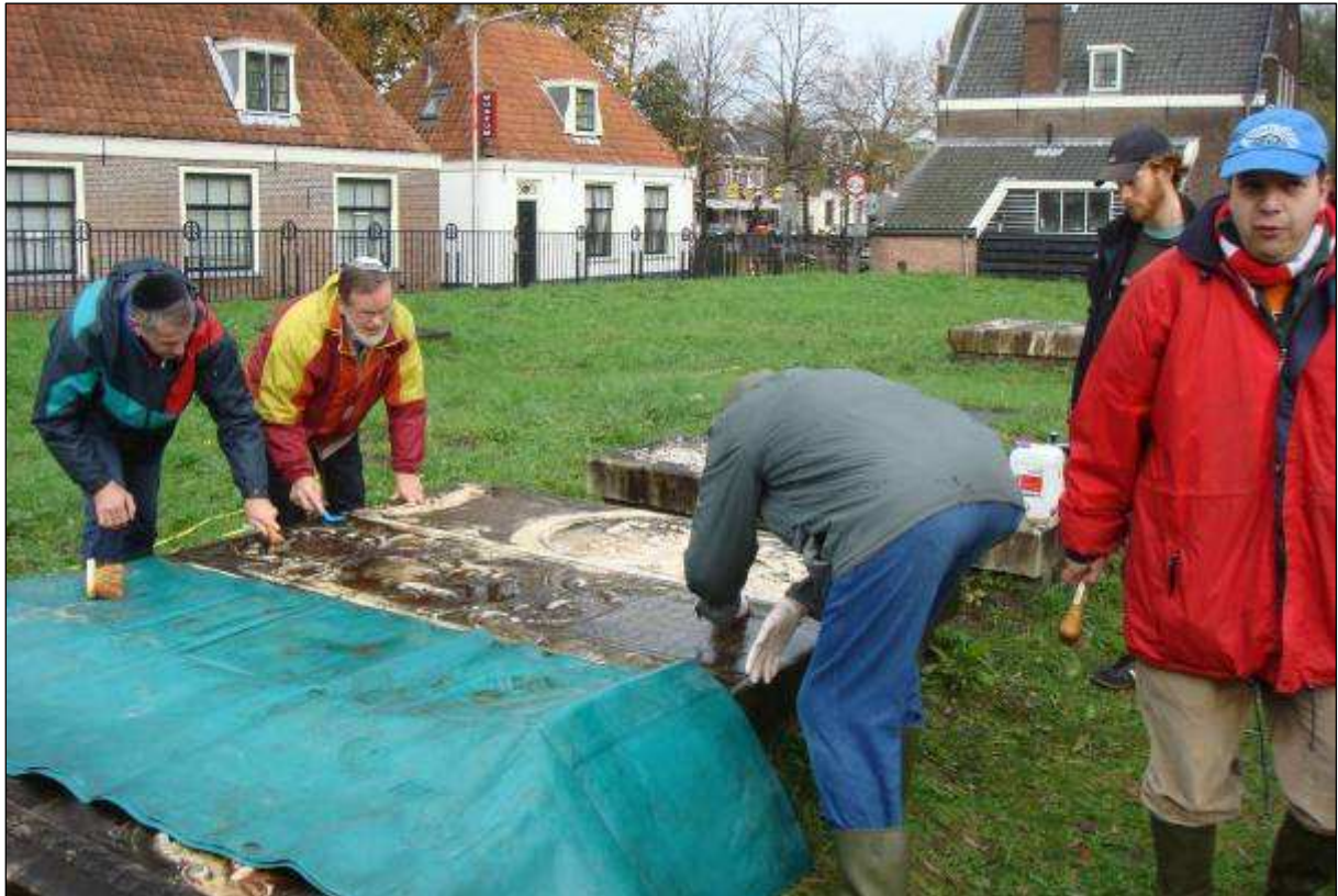
Work in progress at the first test site. To the right caretaker Dennis Ouderdorp.
